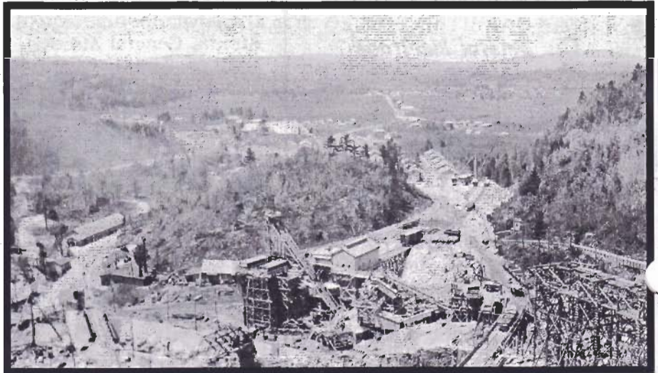
View of Construction Camp and Train Trestle (1927) Hydro-Quebec photo, Gatineau Valley Historical Society (01363)
